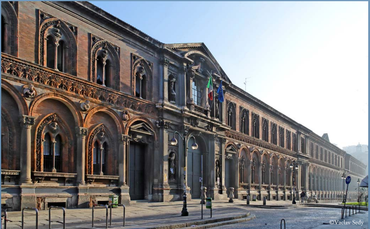
Cà Granda – The main building of the University of Milano
